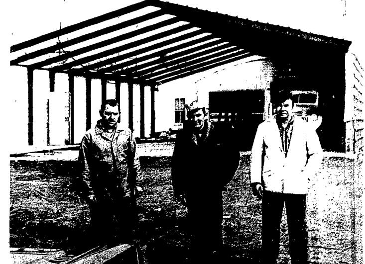
A GROWING INDUSTRY at Hoskins is Hoskins Manufacturing Co. The three owners and workers who put in many hours a day manufacturing as well as erecting the building are (left to right) Richard Doffin, Vernon Delp and Kyle Delp. The size of the new building can be compared with the original plant with the rounded roofline seen through the new steel structure.
